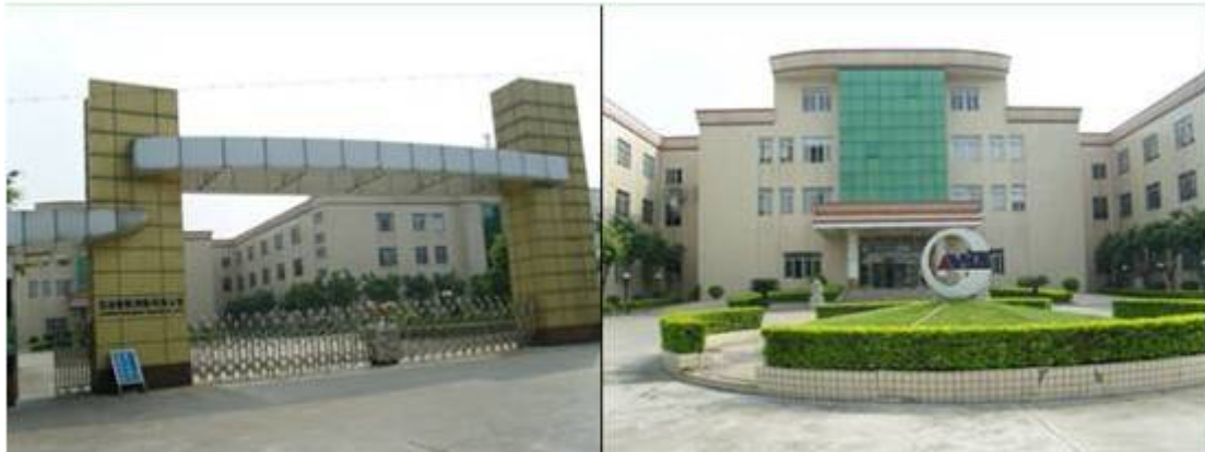
Altrust headquarter building
